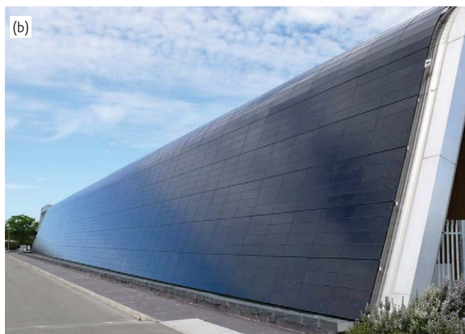
Fig. 2 (a) The 40 kWp facade of the Northumberland building at Northumbria University, UK, which uses the crystalline Si solar modules manufactured by BP Solar (Saturn modules). (b) The 85 kWp facade of the Technium OptIC (Opto-electronics Technology and Incubation Centre) in St Asaph, Wales, which is covered with CIGS modules manufactured by Shell Solar.
