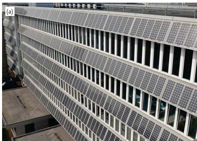
Fig. 2 (a) The 40 kWp facade of the Northumberland building at Northumbria University, UK, which uses the crystalline Si solar modules manufactured by BP Solar (Saturn modules). (b) The 85 kWp facade of the Technium OptIC (Opto-electronics Technology and Incubation Centre) in St Asaph, Wales, which is covered with CIGS modules manufactured by Shell Solar.
