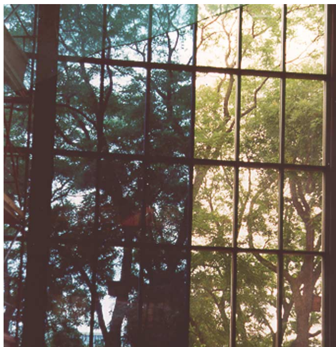
Fig. 3. South facing view of a portion of the 8 x 17 m electrochromic E-Control™ glass made by Flabeg and installed in the Stadtparkasse Dresden am Altmarkt. The left portion of the window is colored. (Source: H. Wittkopf, Flabeg.)
