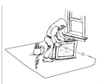
the edges of a door. You can use a plane on friction surfaces such as the edges of windows that rub together when you open or close the window.
